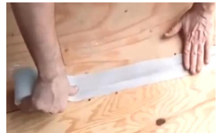
Figure 2: Installing Seam Tape
