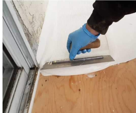
Figure 7: Spreading Base Coat
