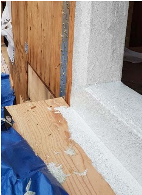
Figure 6 - Waterproofing verticals (door sill)
