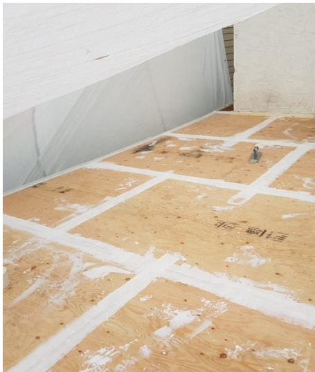
Figure 3: Finished Seam Tape
