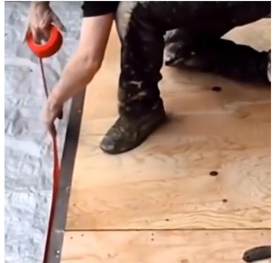
Figure 5 - Installing Red Poly Perimeter tape
