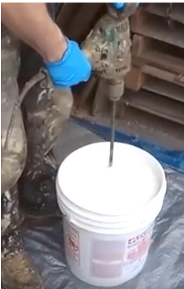
Figure 8: Mixing Base Coat
