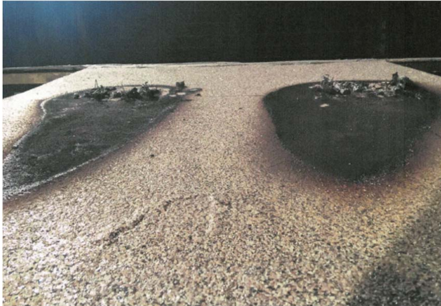
Photograph 3: Class B Burning brand after test. Flexstone Pedestrian Deck Coating System
