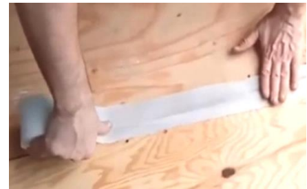
Figure 1: Installing Seam Tape
