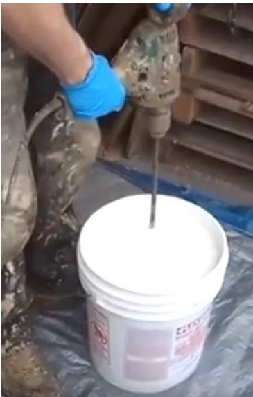
Figure 8: Mixing Base Coat
