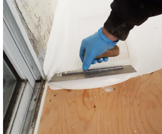
Figure 7: Spreading Base Coat
