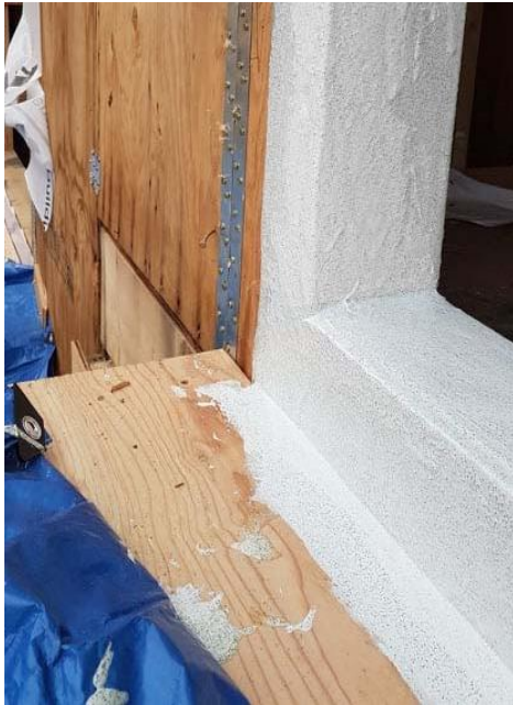
Figure 5 - Waterproofing verticals (door sill)
