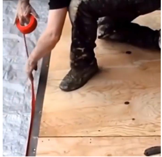
Figure 4 - Installing Red Poly Perimeter tape
