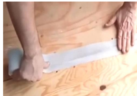
Figure 2: Installing Seam Tape
