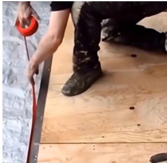
Figure 5 - Installing Red Poly Perimeter tape
